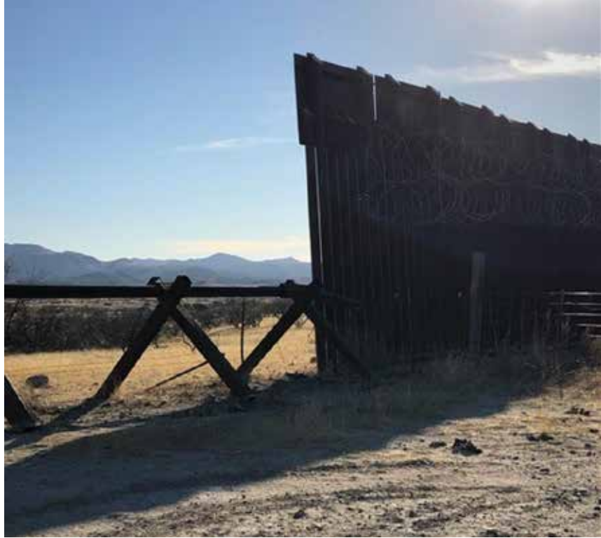
Approximately thirty minutes outside of Nogales, Arizona, the border wall transforms into “Normandy” barricades for several miles. Courtesy: Loyola University Chicago School of Law Immigration Law Practicum
